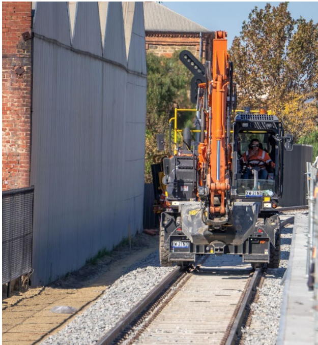
Hi-rail machine on the new passenger rail track (May 2024)
