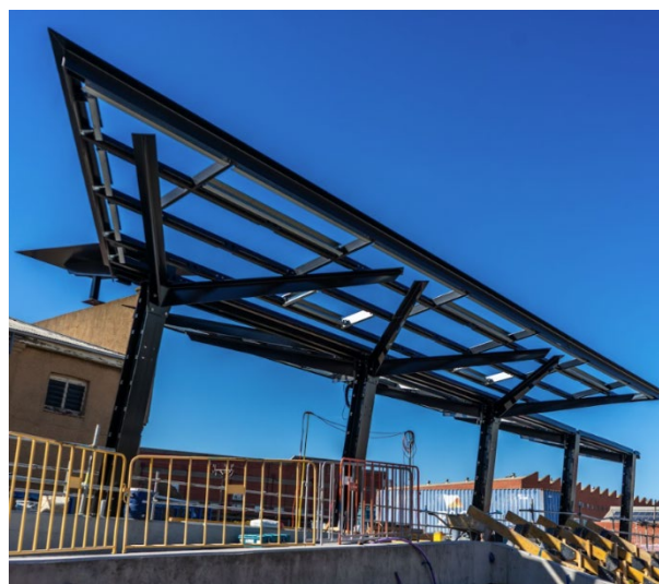
Installed station shelter canopy (May 2024)
